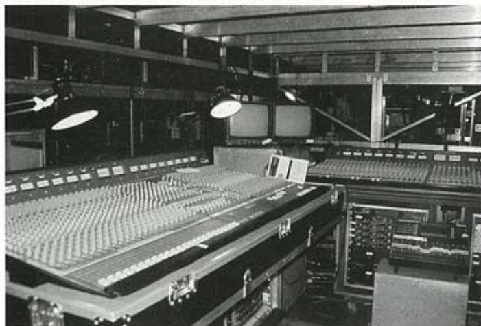
Monitoring desk below stage level.
