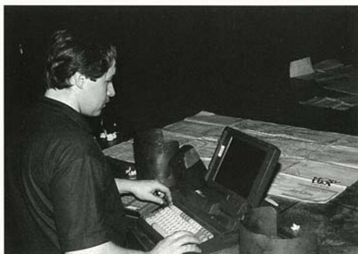
Production electrician Alistair Grant working beside the tin reflected footlights, with the Rosco Lightwright programme on his PC. The Arri portable controller is alongside.
