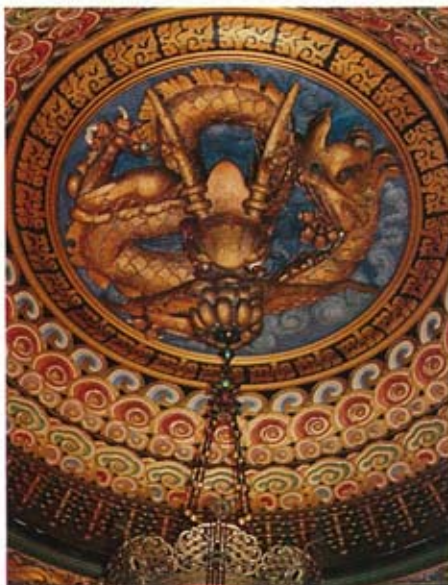
5th Avenue Theatre: The auditorium dome from which a writhing dragon vomits the chandelier.
